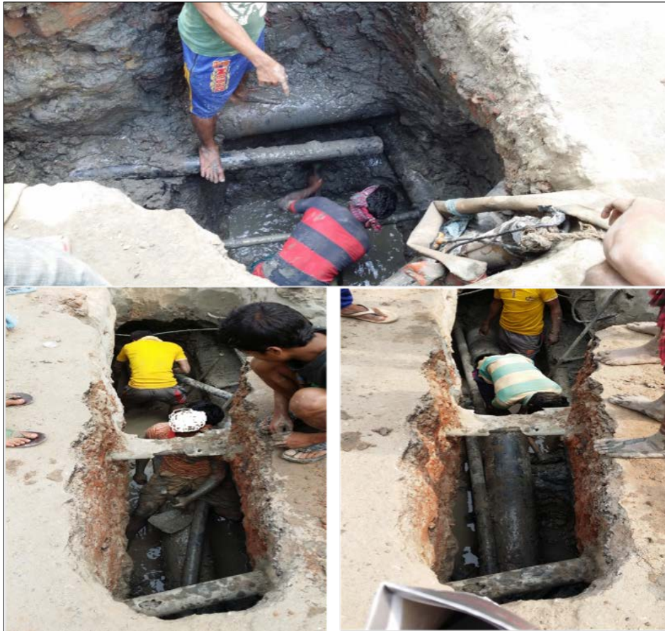
Figure 4.2: Workers working in underground unsanitary sewerage
