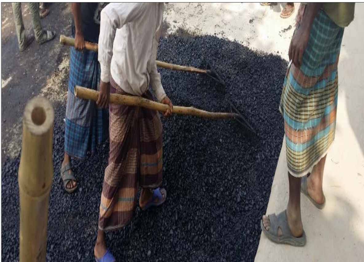
Figure 4.6: Workers making asphalt pavements with hot-lay bituminous materials
