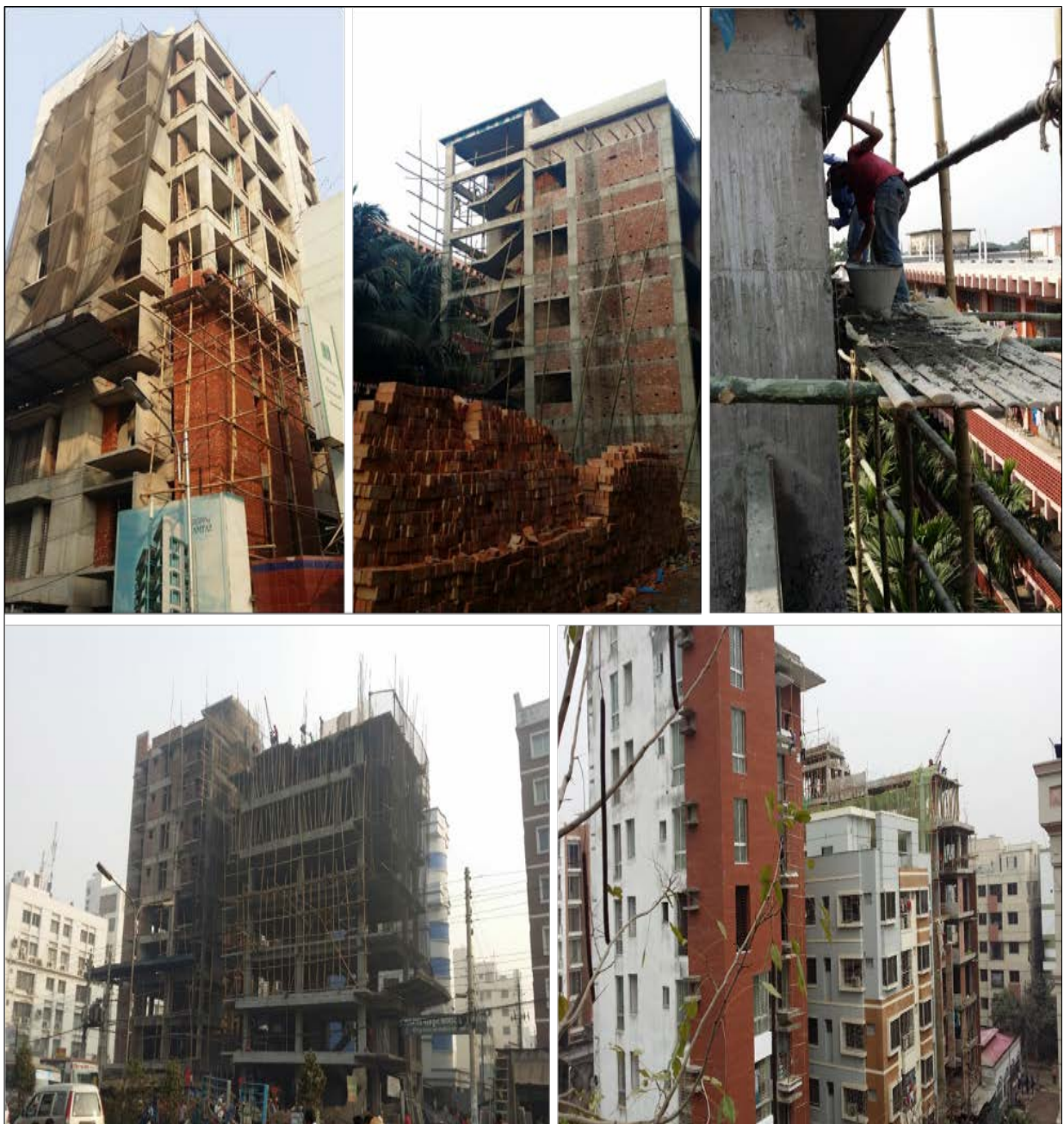
Figure 4.7: Workers working on high scaffolds and ladders made of bamboo
