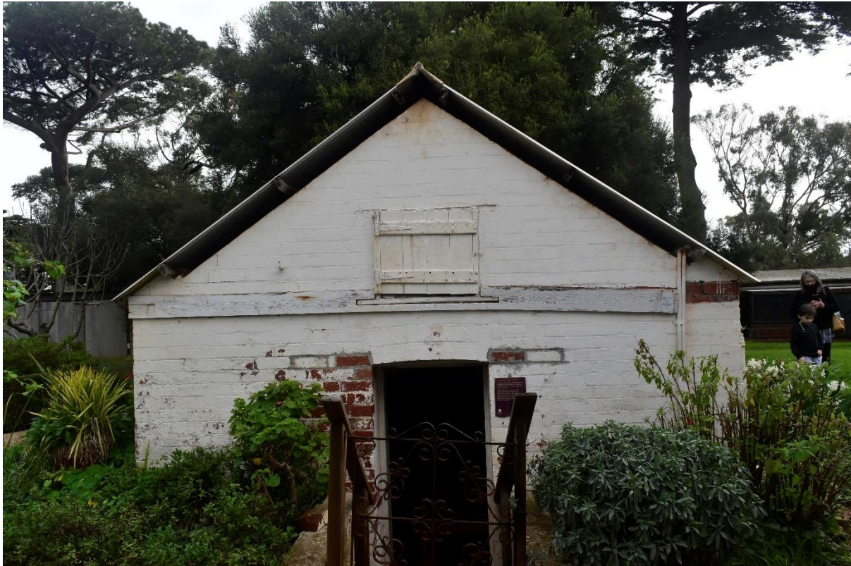
Figure 5.2.2.12 The exterior of the Amess half-cellar. Note the thin plaster or white paint used to cover the bricks (Rünzi 2021).
