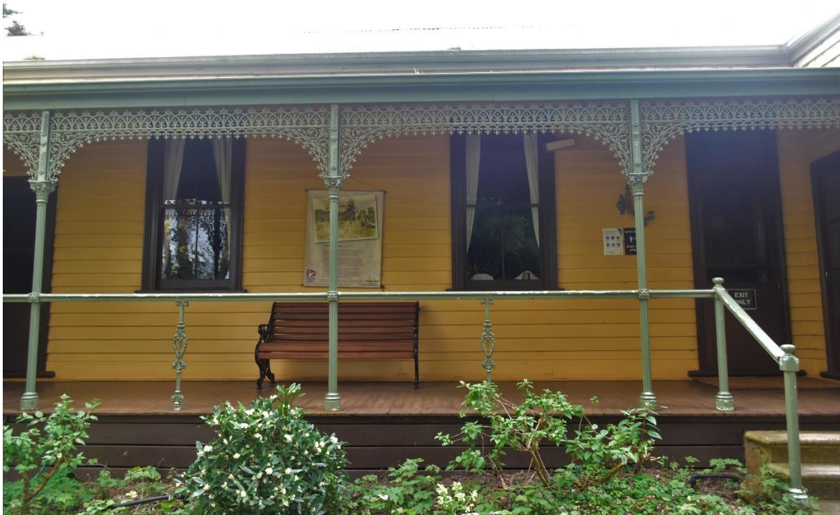
Figure 5.2.2.1 The front façade of Amess House. Note the ornate cast iron verandah decoration (Rünzi 2021).
