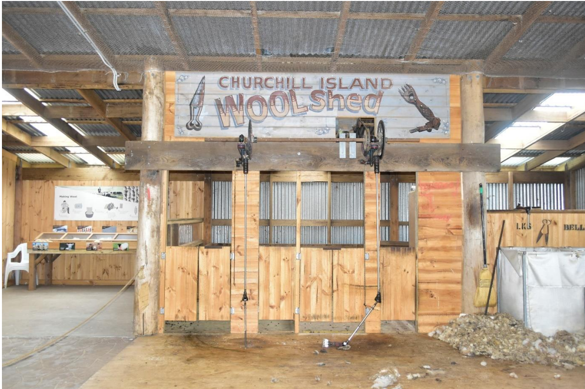
Figure 5.1.1.18 Inside the woolshed built by the National Trust of Australia (Rünzi 2021).
