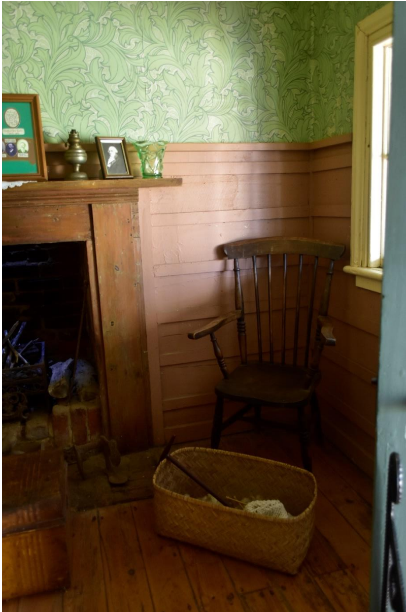
Figure 5.2.1.8 Details of the flooring and wall in the southern Rogers' Cottage (Rünzi 2021).
