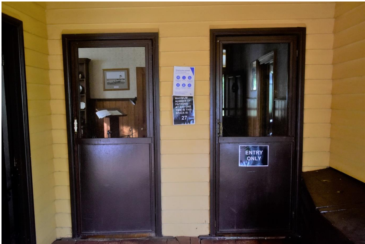
Figure 6.6.2 The doors of Amess House. Fly screen covers the top half of the door, allowing for extra light and airflow through the house (Rünzi 2021).
