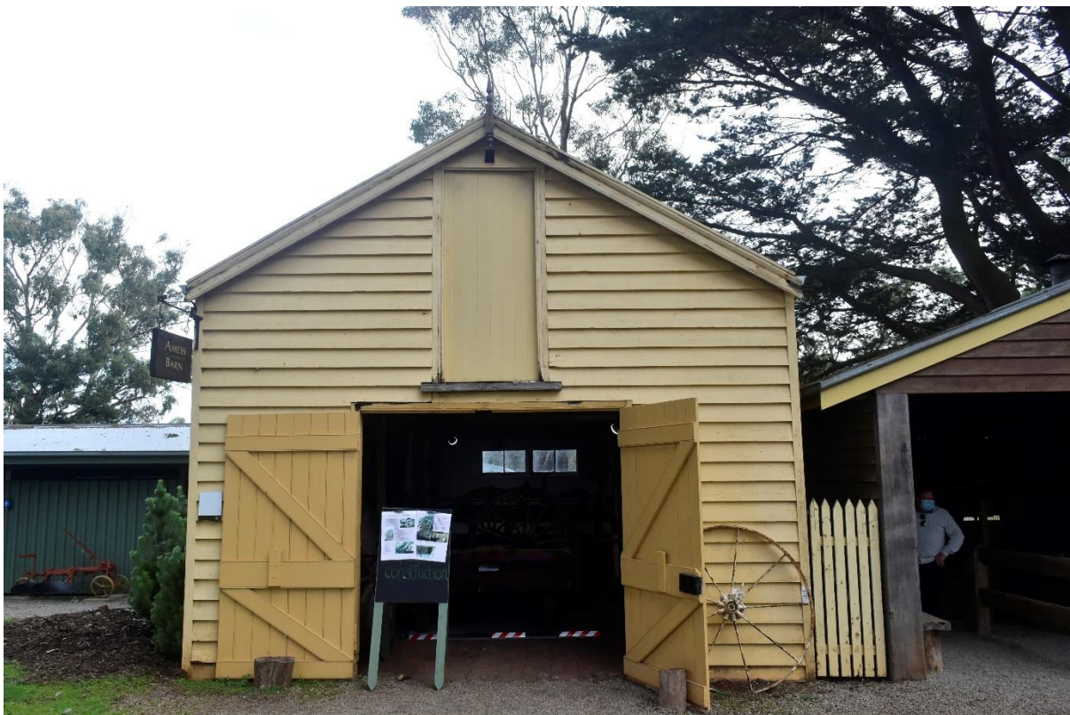
Figure 5.2.2.11 The exterior of Amess Barn. Note the zigzag bracing on the barn doors (Rünzi 2021).
