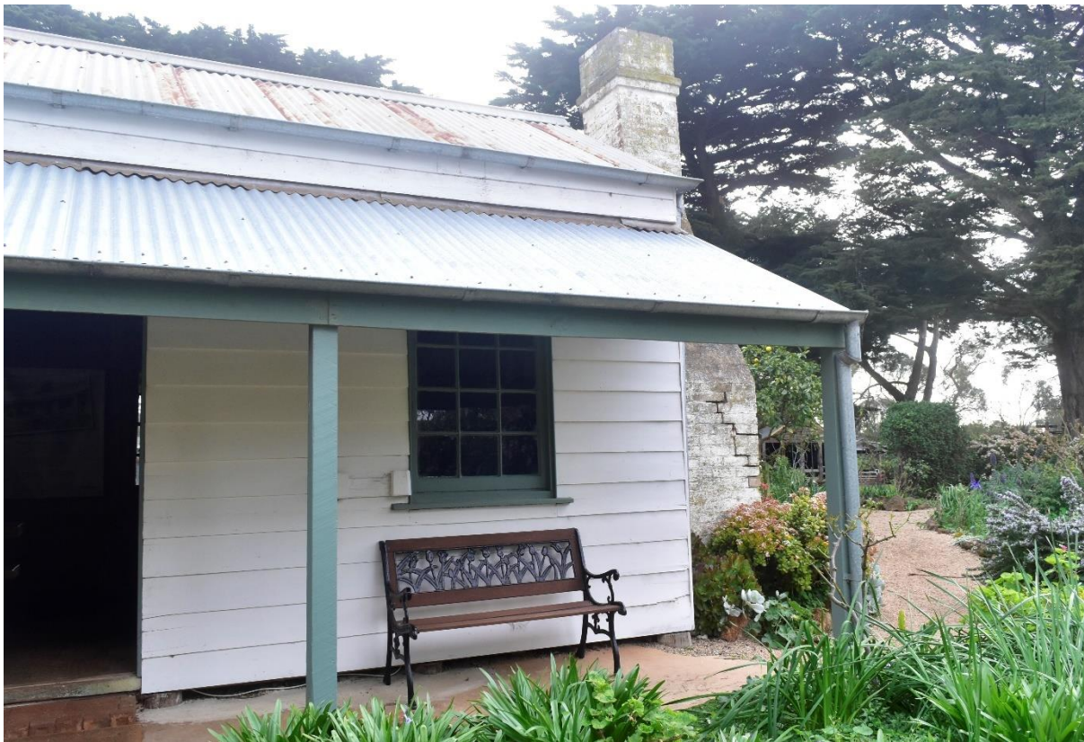
Figure 5.2.1.1 External façade of the northern Rogers' Cottage. Note the fresh paint applied to the wooden slats and beam, the tree stumps upon which the cottage is propped up on the right, and the chimney on the far right of the building (Rünzi 2021).
