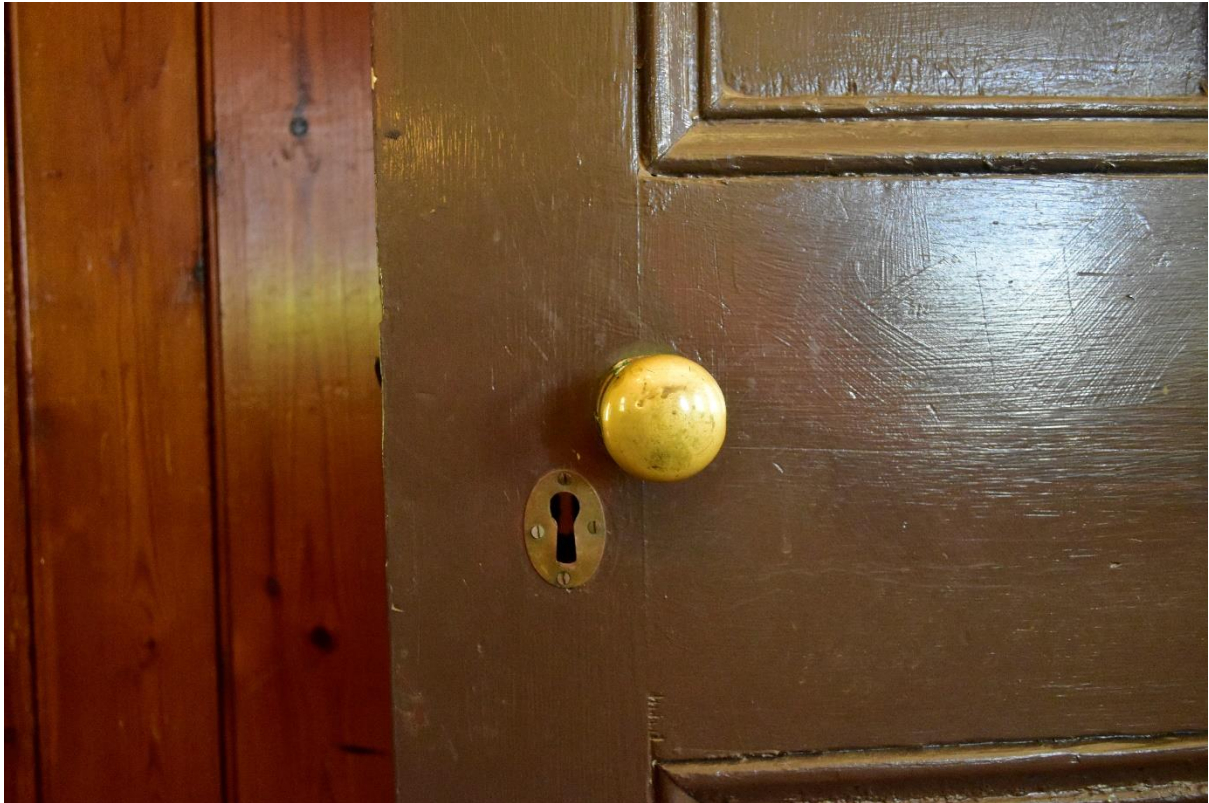
Figure 6.6.3 An example of the older locking system in Amess house, a keyhole cut into the doorframe (Rünzi 2021).
