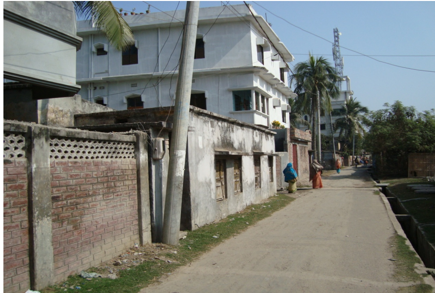
Photo 3: Pucca houses on the western side of Alampur (Study CDC 1).
