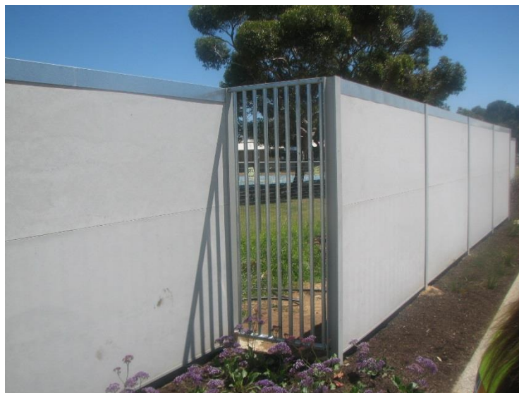
Figure 22. Visual connection between schools, afforded in discrete locations.
