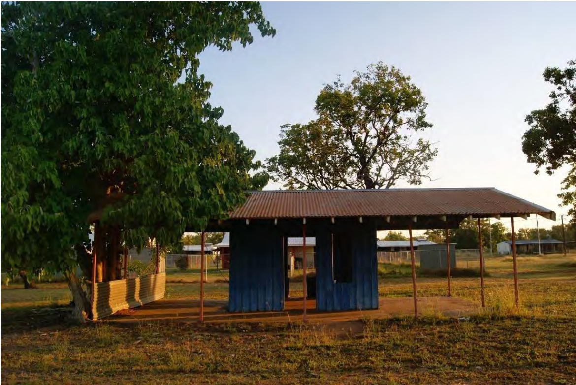
Figure 4.2 North aspect of Econo Hut 3 (Photograph: Elspeth Hodgins 23/04/2022).
