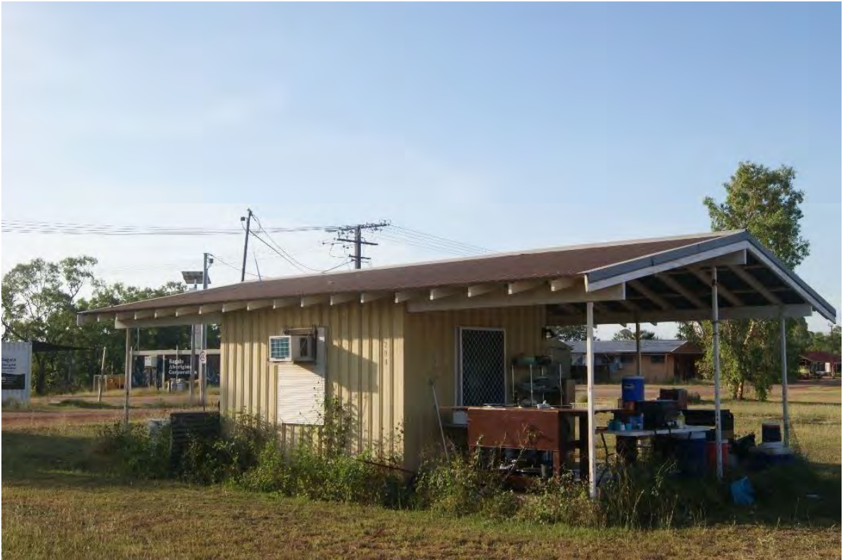
Figure 3 Southeast aspect of the renovated Econo Hut (Photograph: Elspeth Hodgins, 23/04/2022).
