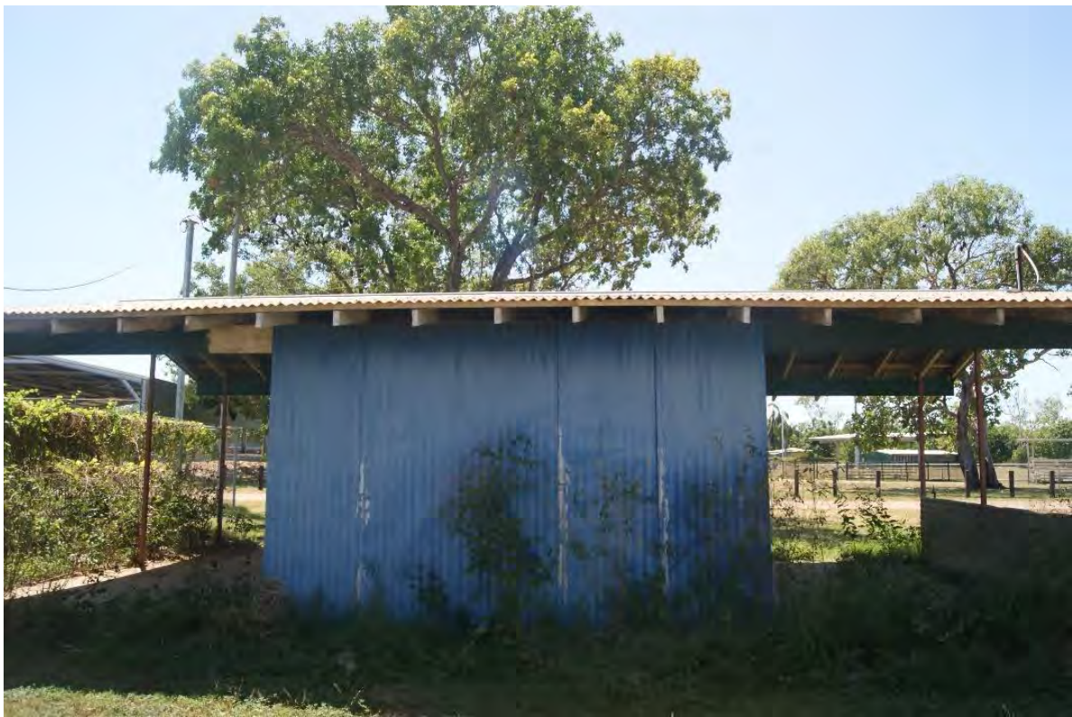
Figure 1 Southern aspect of Econo Hut 1 (Photograph: Elspeth Hodgins, 23/04/2022).
