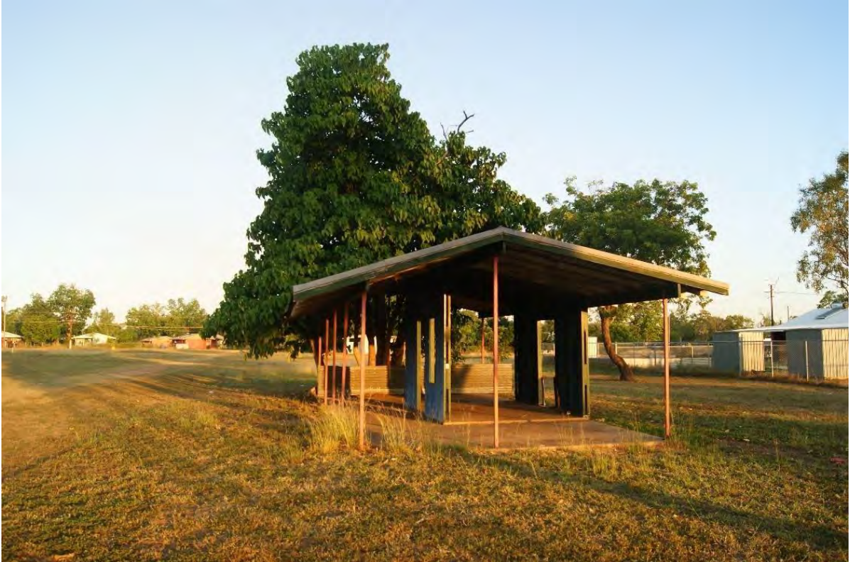
Figure 2 Western aspect of Econo Hut 3 (Photograph Elspeth Hodgins, 23/04/2022).
