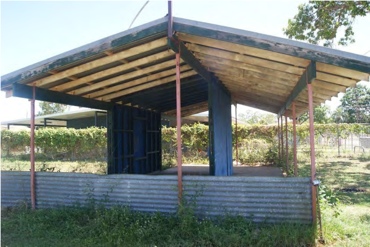
Figure 2 Eastern aspect of Econo Hut 1 (Photograph: Elspeth Hodgins, 23/04/2022).
