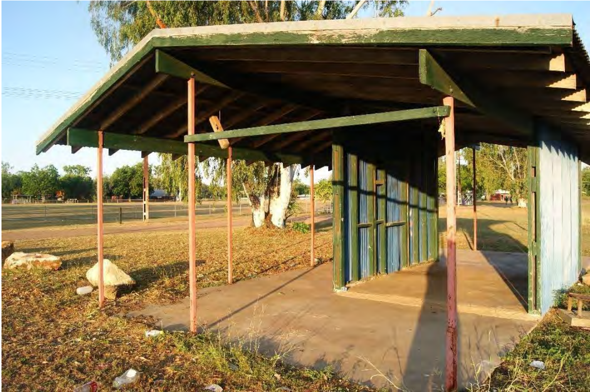
Figure 1 Western aspect of Econo Hut 2 (Photograph: Elspeth Hodgins, 23/04/2022).
