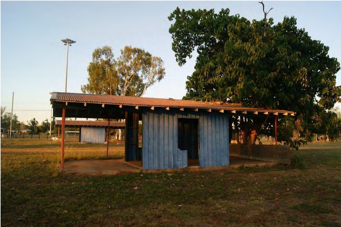
Figure 3 Southern aspect of Econo Hut 3 (Photograph: Elspeth Hodgins, 23/04/2022).
