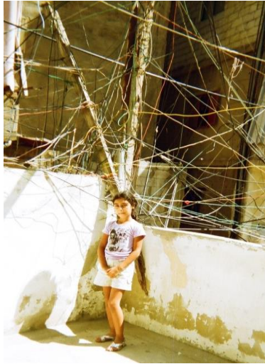
Figure 27: Taken by an elderly refugee on her family’s roof, showing the dense network of electrical wiring and water piping (thicker black strands) (201, photograph 8)
