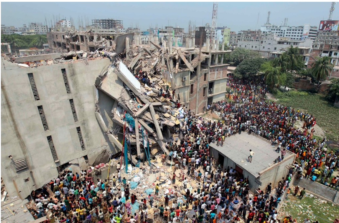
Figure 5: Rana Plaza Collapse 2013
