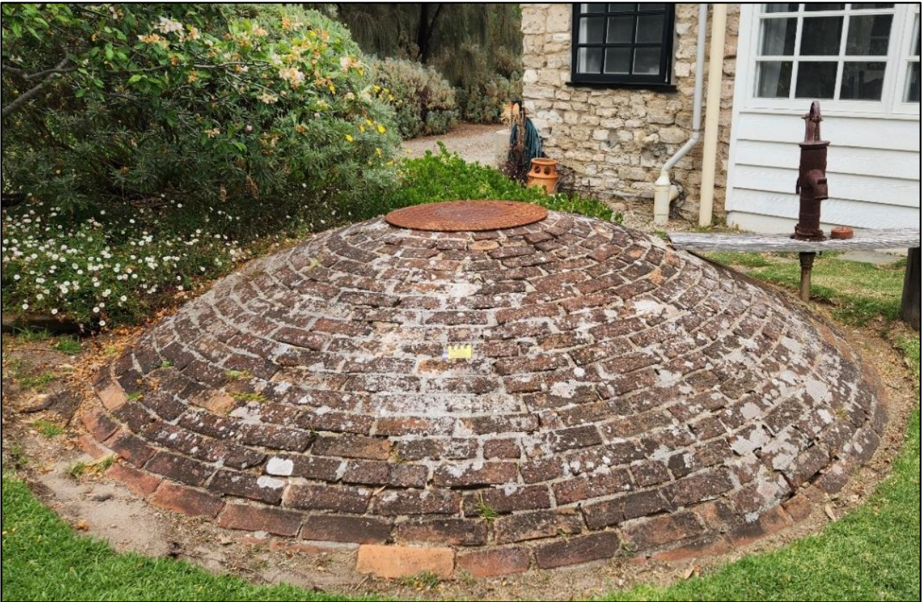
Figure 16. Water well behind the Fountain Inn said to be constructed from bricks salvaged from the Solway shipwreck (Image by author)
