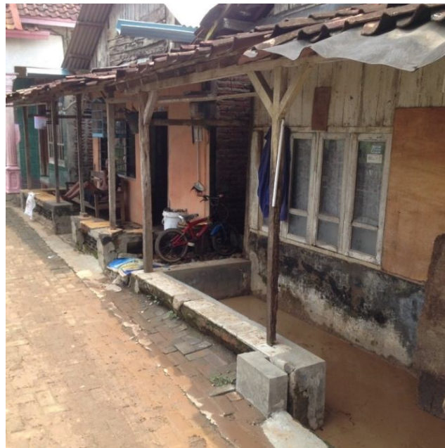
Figure 8-5: Mangun Harjo settlements covered with mud after the flood receded, Semarang, Indonesia, in February, 2016
