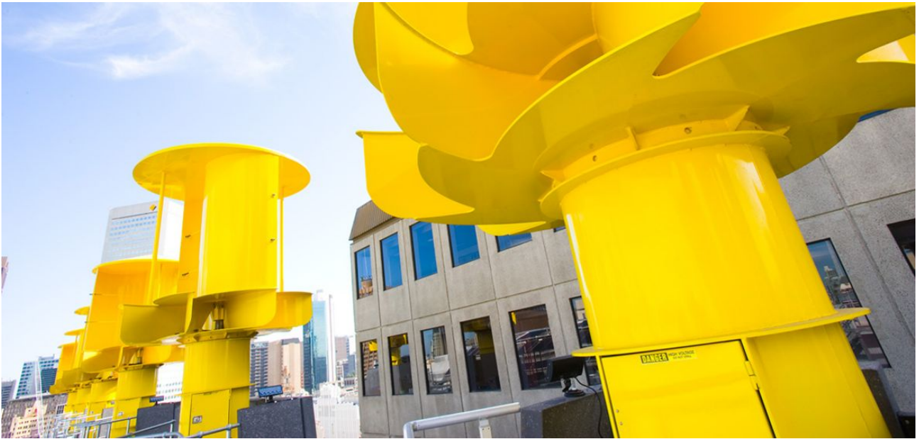
Figure 7. CH2's roof mounted wind turbines (Hansen Yuncken 2017, n.p.)
