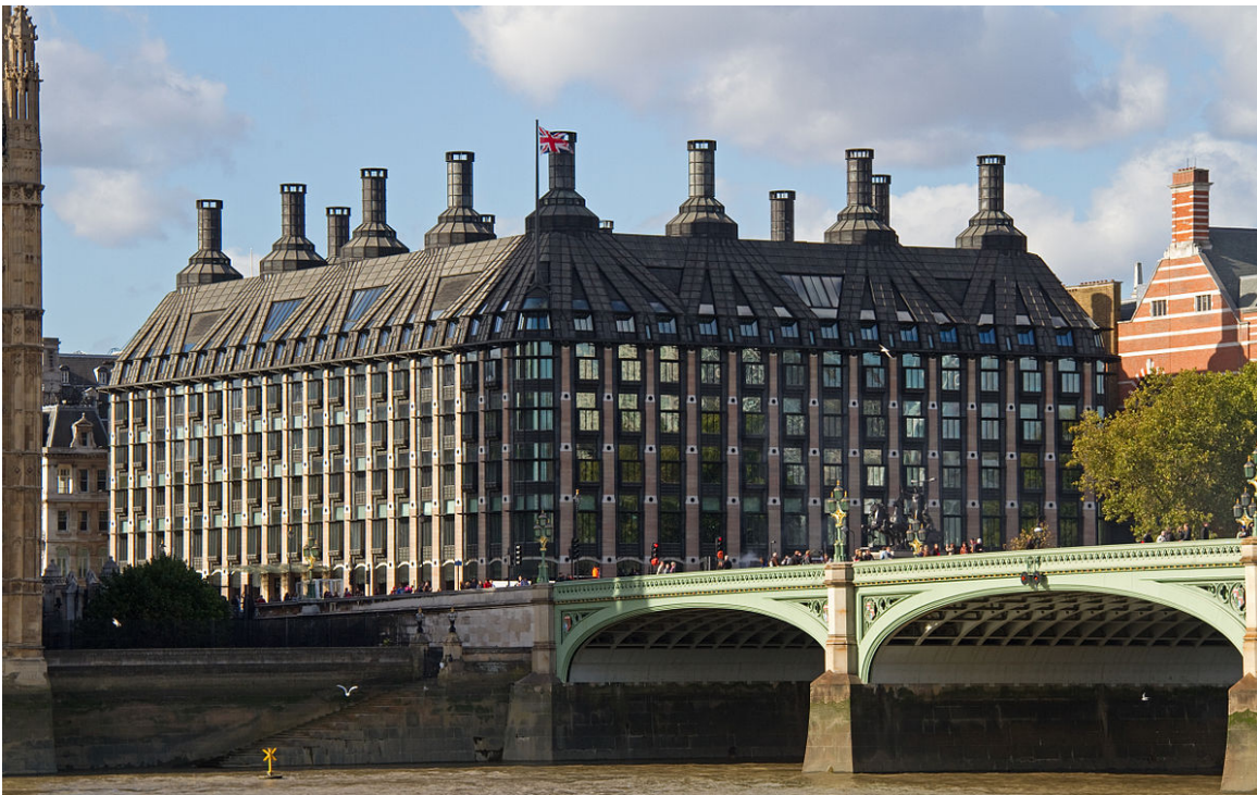
Figure 17. Portcullis House, London (Hisgett 2011, n.p.)
