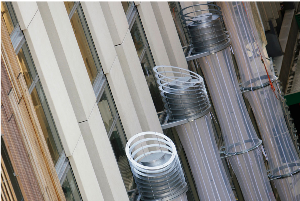
Figure 8. CH2's Shower Towers (City of Melbourne 2017, n.p.)
