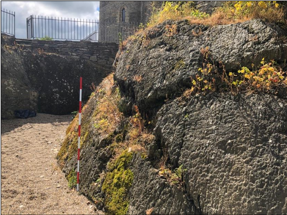
Figure 38. The rock cut motte on the southern side of the castle facing west.
