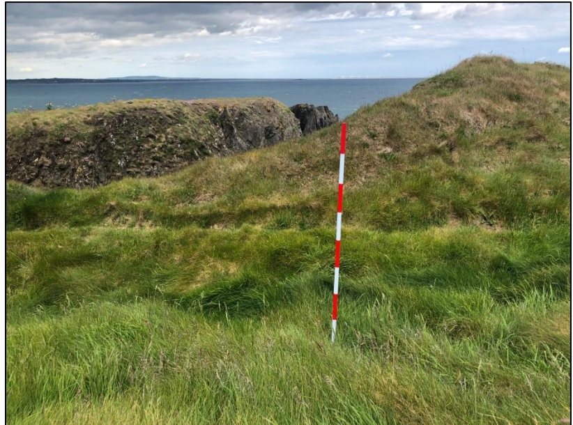
Figure 1. Section of the broken earthworks at Baginbun.
