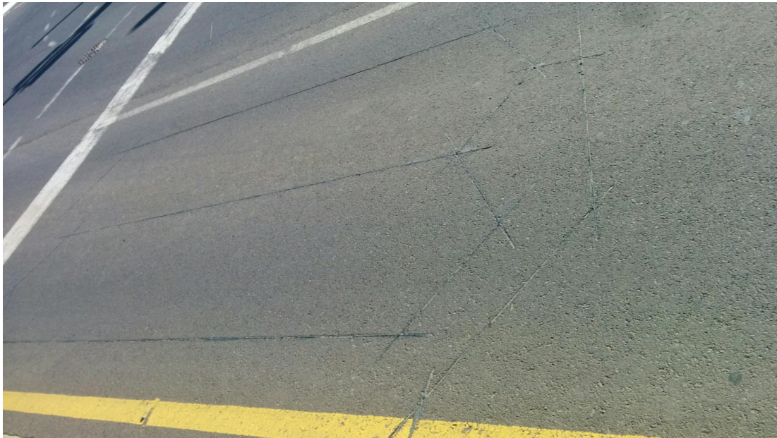
Figure 2.1: Close up photograph of loop detector showing the outline of the loop
