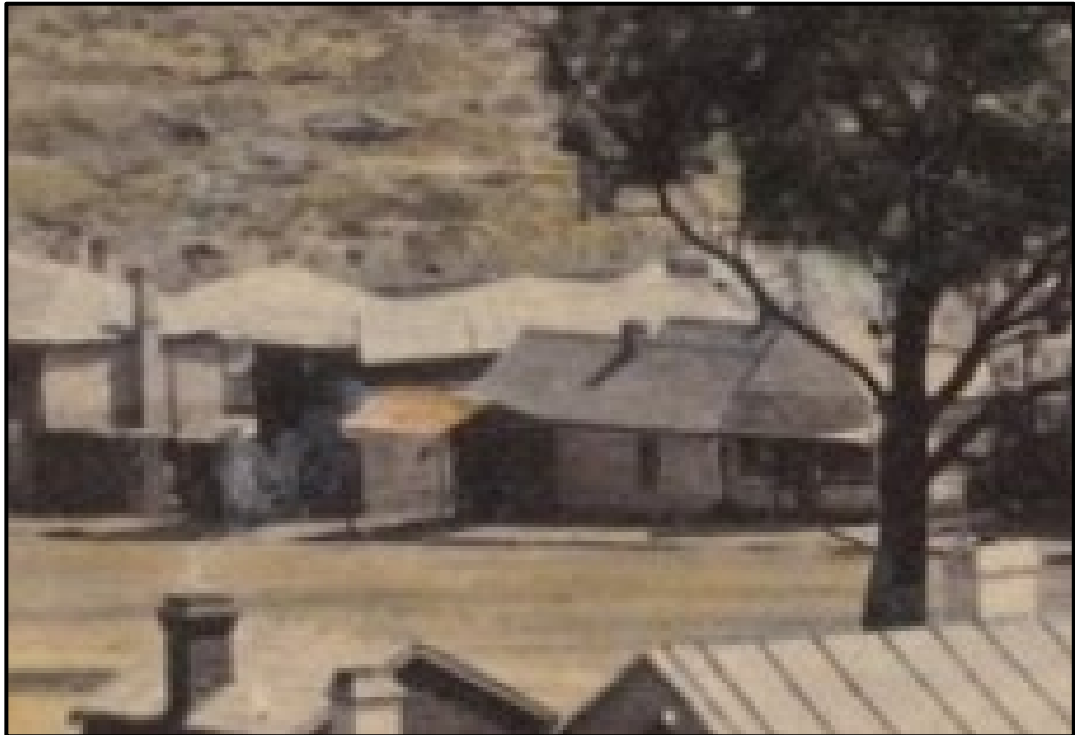
Figure 5.3: Fanny Finch's Restaurant, Castlemaine, c1859. 103
