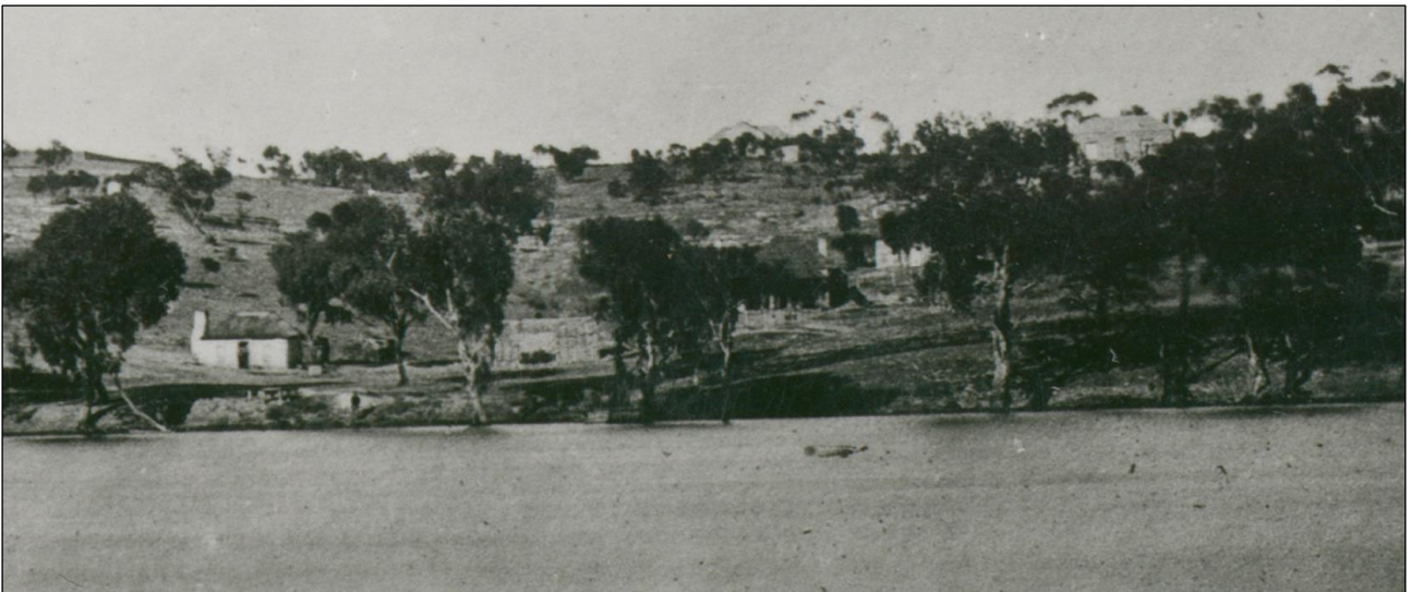
Figure 6: Buildings at Blanchetown, c.1870–1872; description reads “customs cottage (near river), police station (partly hidden by trees)” Source: Anon. c.1870–1872, Blanchetown Collection, State Library of South Australia also appears in the Ewens Collection, State Library of South Australia.
