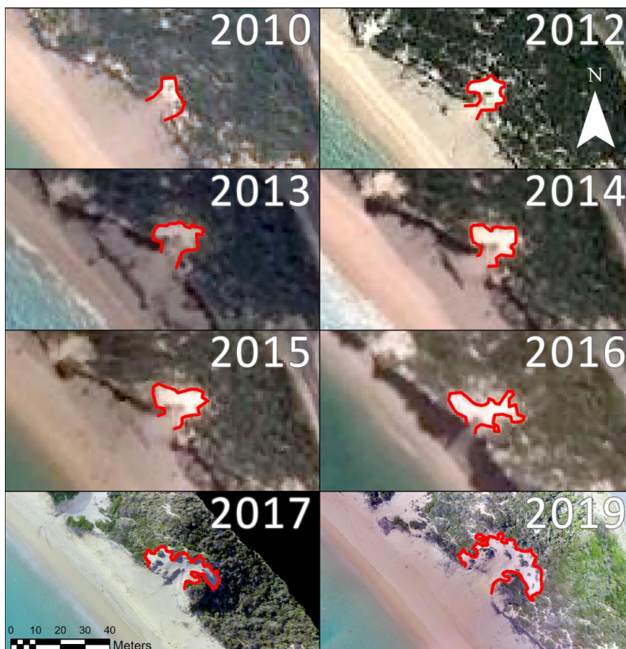
Figure 47: Georectified historical aerial imagery of the growth of the blowout. The blowout has expanded between 2010 and 2019.
