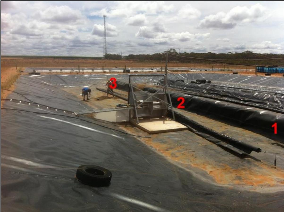
**Plate 6.2.** The emptied and cleaned Flocculation high rate algal pond (HRAP) at the Kingston on Murray wastewater treatment system, Australia, prior to the transfer of the Wastewater Treatment HRAP effluent. The location of the three sampling points (1-3) used to determine the efficacy of flocculation are also shown.
