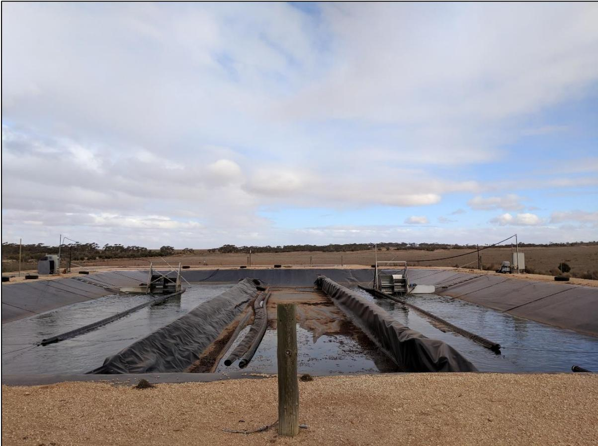
**Plate 2.1.** The high rate algal ponds at Kingston on Murray Wastewater Treatment Plant (Kingston on Murray, Australia)
