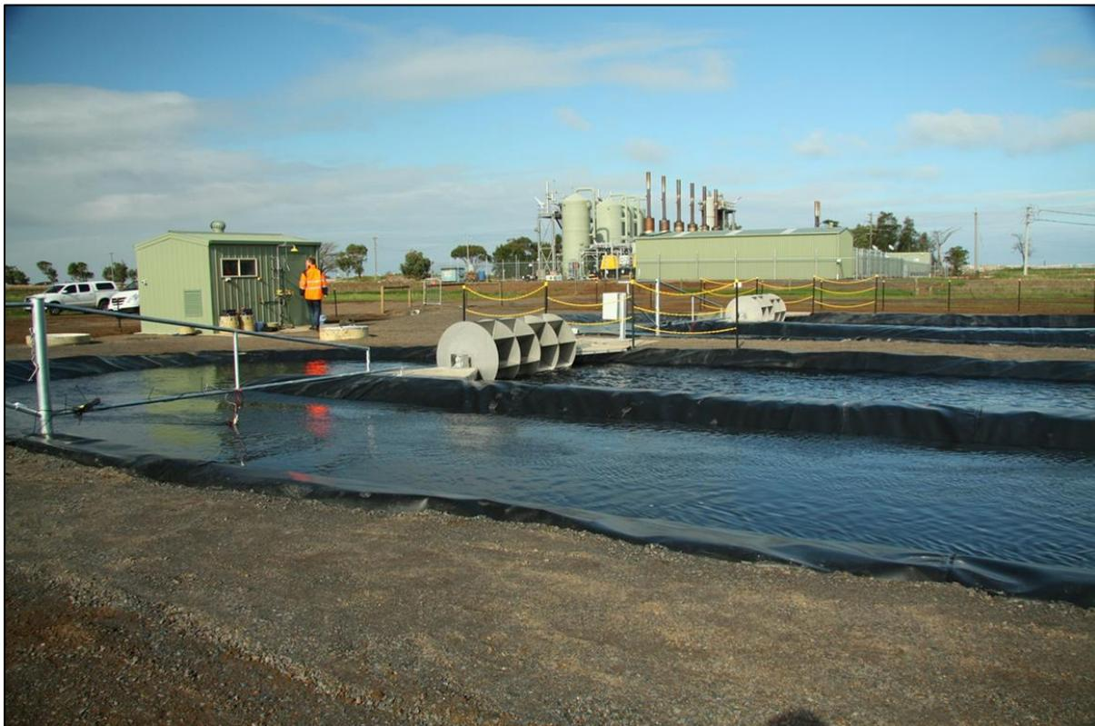
**Plate 1.2.** Two high rate algal ponds at Melbourne Water Western Treatment Plant, Werribee, Australia, fed anaerobic and facultative lagoon treated domestic wastewater.
