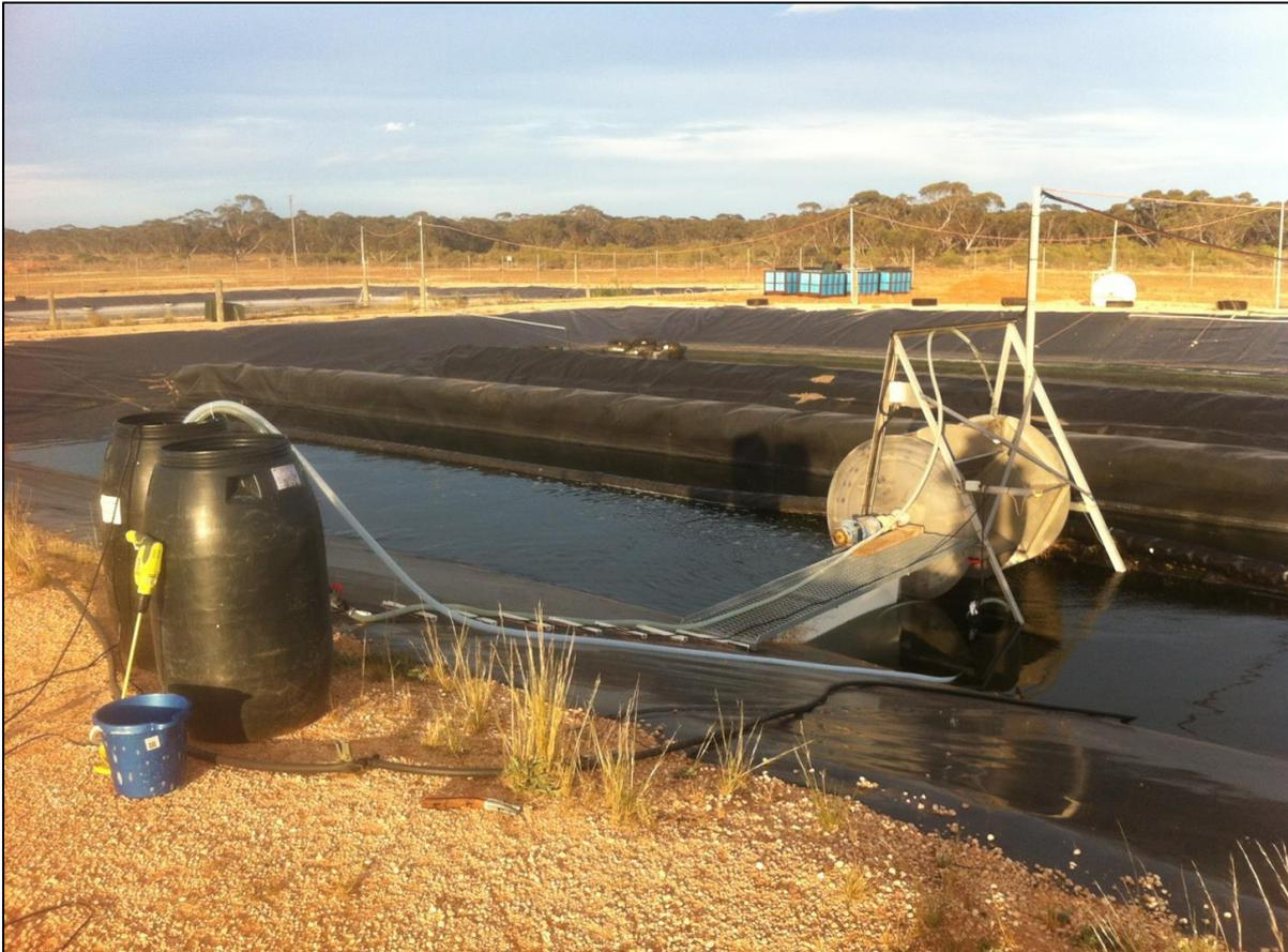
**Plate 6.1.** The dosage apparatus used to add magnesium chloride and slaked lime to the Flocculation high rate algal pond (HRAP) at Kingston on Murray wastewater treatment system, Australia. Also pictured is the paddlewheel in the Flocculation HRAP that was used for mixing after chemical addition.
