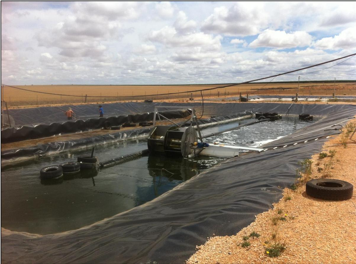
**Plate 6.5.** The Wastewater Treatment high rate algal pond at the Kingston on Murray wastewater treatment system, Australia.
