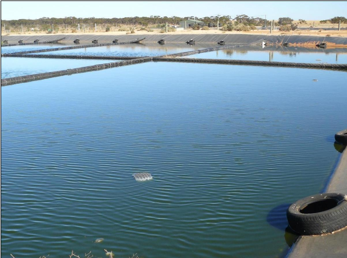
**Plate 1.1.** The facultative waste stabilisation pond at Kingston on Murray wastewater treatment plant, Australia.
