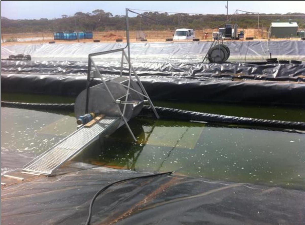
**Plate 6.4.** Visible flocculation and sedimentation of the microalgae biomass in the Flocculation high rate algal pond at the Kingston on Murray wastewater treatment system, Australia, post-autoflocculation via magnesium hydroxide. The plinth the paddlewheel is mounted on was clearly visible.
