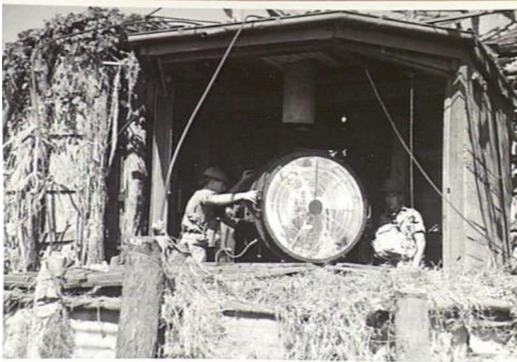
Figure 4-9: Photographs of WW2 search lights. Upper from Flinders NSW and lower Darwin NT. The upper shows the camouflage netting and there are the steel loops in the concrete wall. Darwin's has a wooden shelter rather than concrete. It is expected Juno Point had similar roofing.
