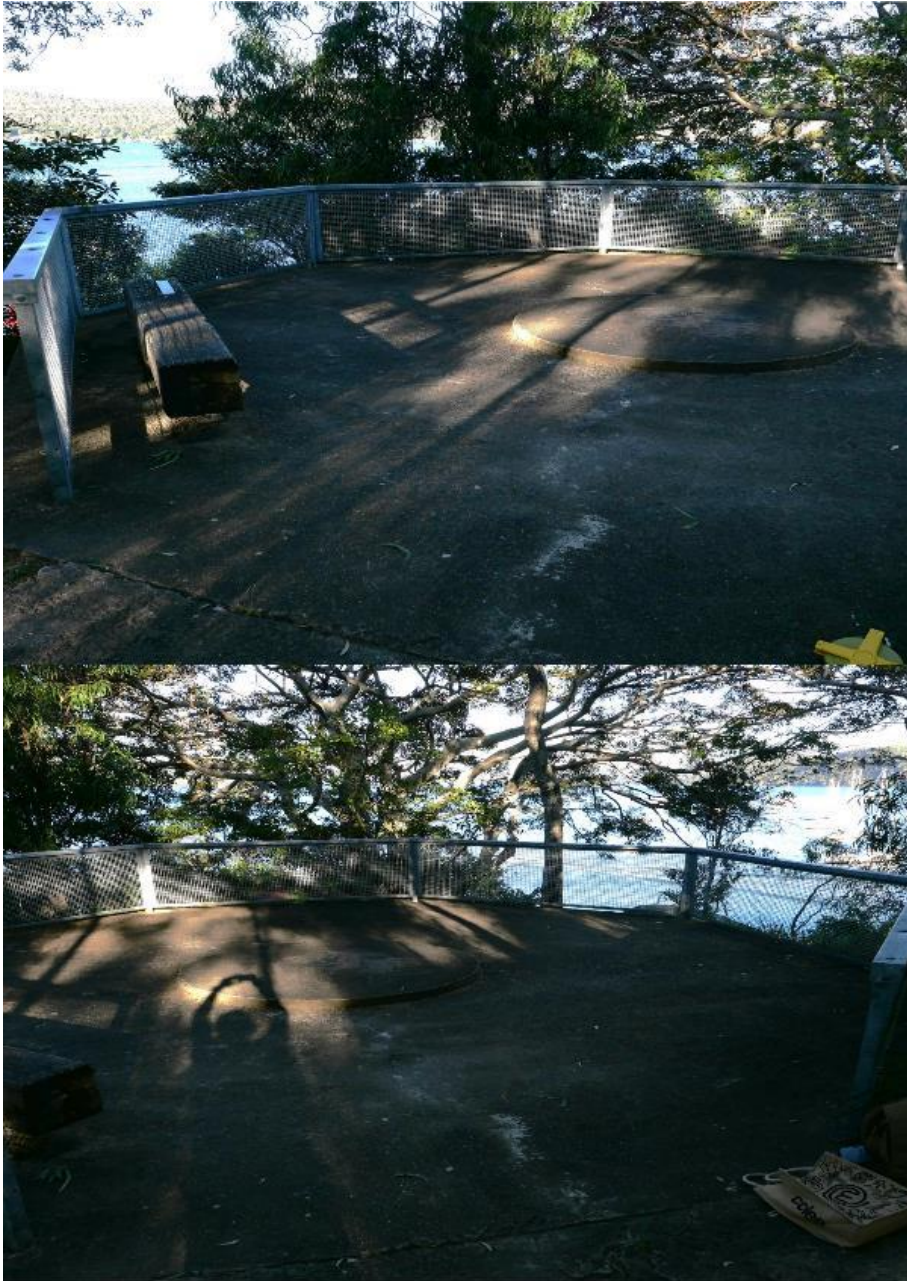
Figure 4-15: Gun position with modern safety barriers installed. The pin in the centre has been replaced brass capping plate flush with the concrete. The round inner circle is the same diameter as Juno Point within 10cm.
