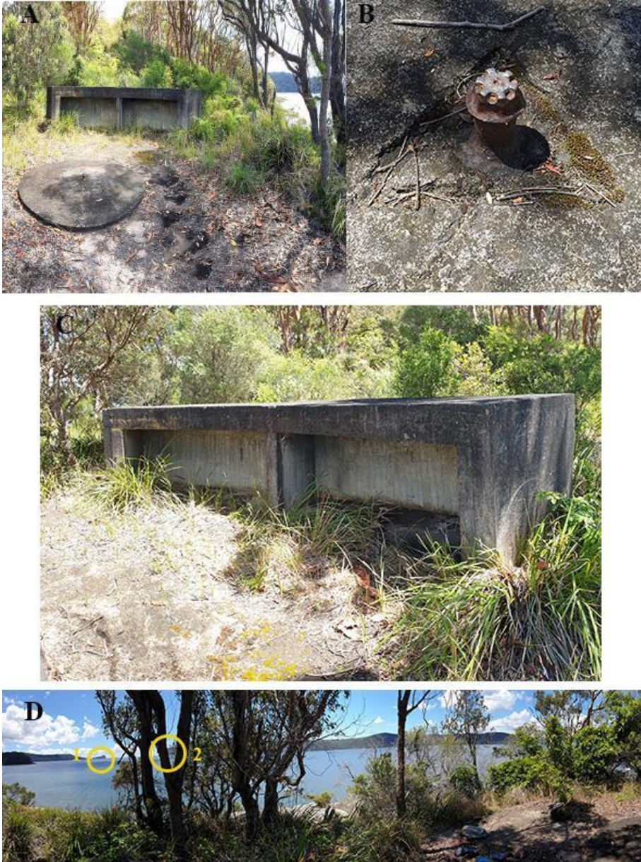
Figure 4-1: Gun position 1 situated near the point of Juno Point. A- Overview of the gun position and storage bunker. B- Close-up of the centre-notch pin with a possible survey mark. C- Ammunition storage bunker. D- View from the gun overlooking Broken Bay to the e east. 1- Lion Island. 2- Barrenjoey Head.
