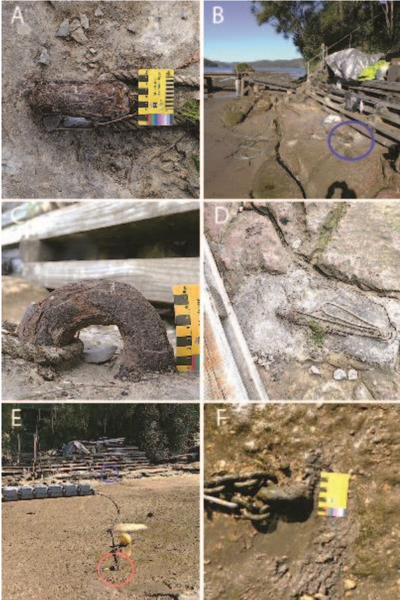
Figure 4-21: Close up of the securing rings with associated sizing. Securing ring F is only above water a very low tides. Photograph D shows a large amount of concrete around the shore ring, with diameter and depth of each hole unknown. There was a gate on the northern boom.
