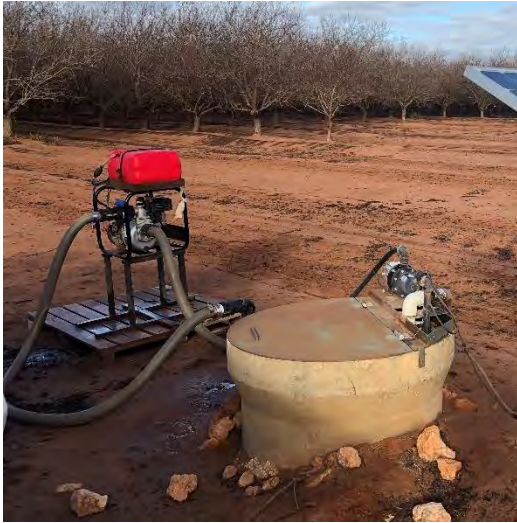
Figure 4-6: One of the shallow drainage pits in the Alma Almond Orchards.
