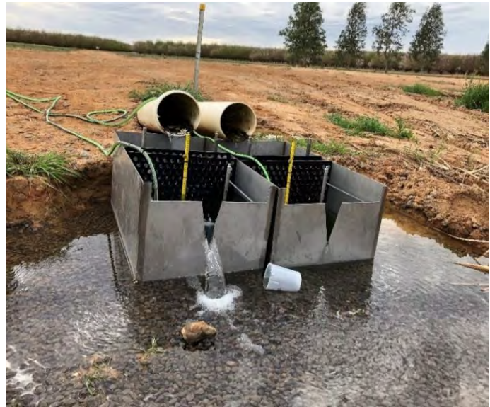
Figure 4-5: Discharge outlet pipes and the installed V-notch weirs as part of the study.
