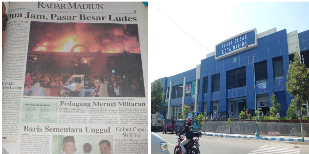
Figure 6.1 Madiun Central Market: Fire and after Renovation
