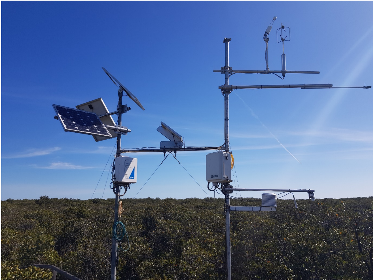
Figure 2: MEP and EC equipment installed at St Kilda Mangrove Trail
