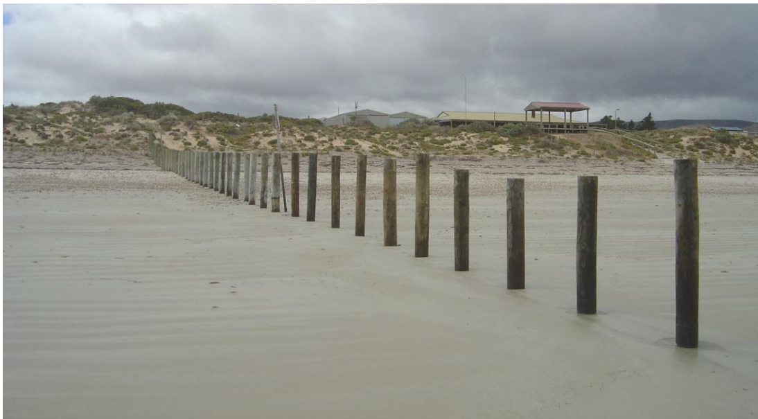
Figure 1.4b: Bollards at Aldinga
