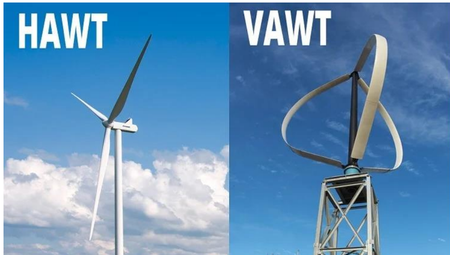
Figure 1 – Difference between Horizontal & Vertical Axis wind turbines in construction
